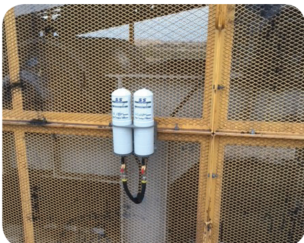
Lubrication system mounted on the outside of a safety cage of a conveyor application.
